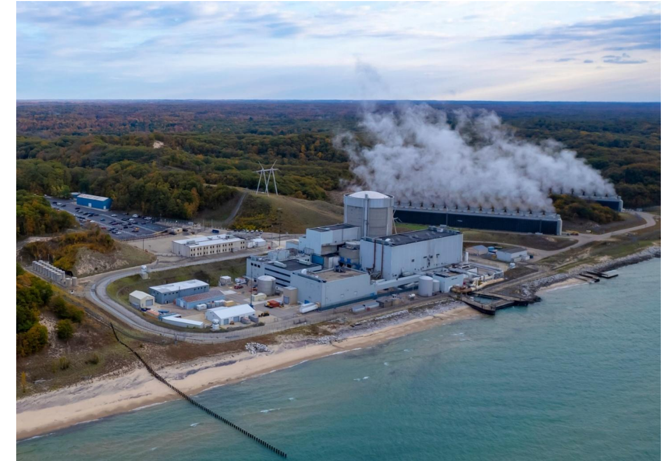
Palisades Nuclear Power Plant
